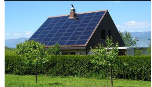
Example of a Solar Conversion System, Structure-mounted
